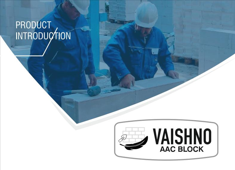
V-Lite AAC blocks are a lightweight Autoclaved Aerated Concrete Block is used as a substitute for conventional building masonary. It is suitable for multistoried structures as it is lighter than standard size bricks and blocks as it is widely accepted globally because of its beneficial proper ties such as lightweight, thermal, sound insulation, fire resistant, low capillary water absorption, easy to cut, and other benefits which ease the process of construction.
